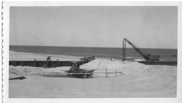
Figure 5. Construction of Jetty – Photo by Wilbur Corkran 1958.
