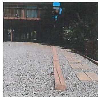
Figure 1: Paver Pathway More and more residents are choosing to use pavers or gravel, which allow infiltration, instead of traditional concrete for driveways and walkways.
