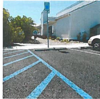
Figure 1: The Delaware CIB's main office located along the Indian River Bay. Their porous asphalt parking lot helps disperse water during high rain events.
