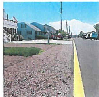
Figure 1: The Town of Fenwick Island installed an infiltration trench along Bayard Street to filter and store stormwater before draining to the canal.
