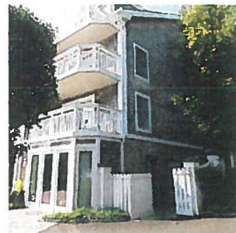
Figure 1: Canalfont Inn in Lewes has a system of drainage pipes that convey water from the roof to planted beds around the hotel.
