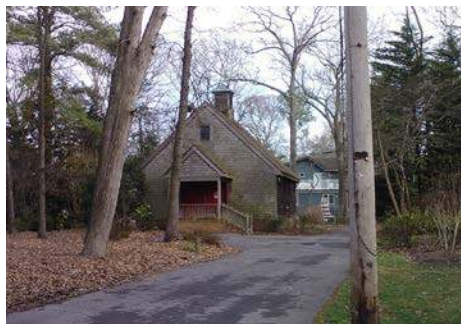
Henlopen Acres Water Plant
